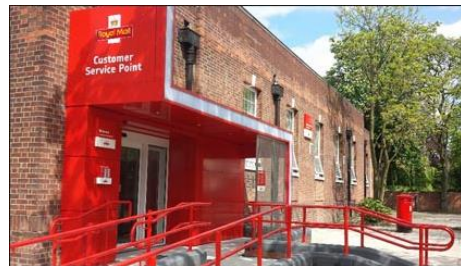
Post sorting office
